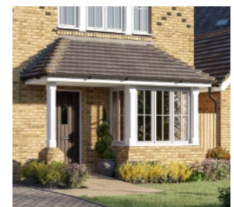
Hipped porch roof
