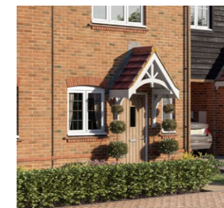
Gable porch entrance
